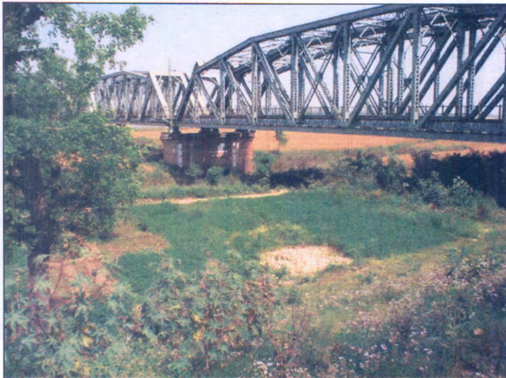
Plate 3 : Satluj River at Phillaur (Below railway bridge)
