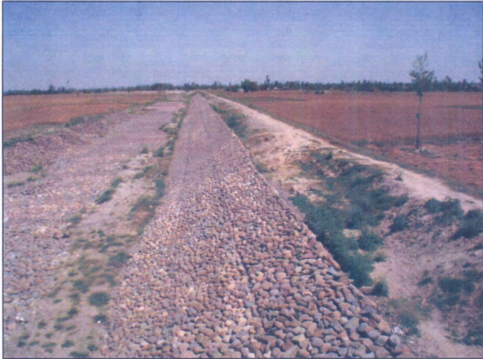
Plate 5 : Embankment along Satluj River at Ludhiana
