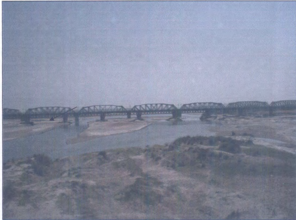
Plate 1 : Satluj river at Phillaur (Railway bridge)
